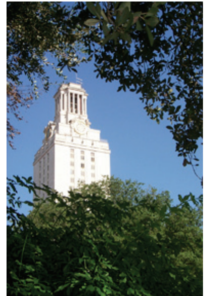
Main Building - "The Tower" Home of the Graduate School in suite 101 (2nd floor)
