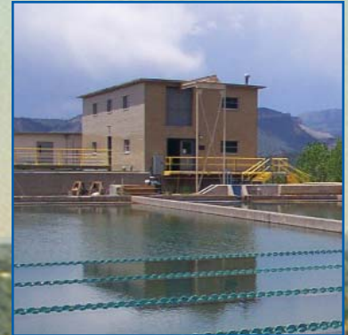
WTP Sedimentation Basins, Durango, Colorado
