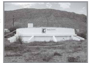
Completed water tank in Manuel Benavides, Chihuahua, Mexico
