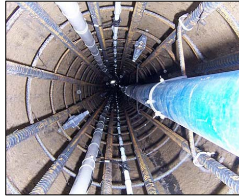
Figure 7: Instrumented Cage During Installation
