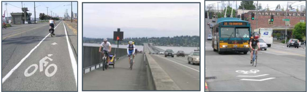
2 3 4 5 6 7 8 9 10 11 12 13 14 15 16 17 18 19 20 21 22 23 24 25 26 27 28 29 30 31 32 33 34 35 36 37 Figure 1: Roadways with Bike Lanes, Separated Bicycle Facilities and Sharrows (Seattle Department of Transportation 2007)
