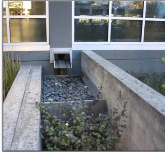
Figure 3-4: Downspout directed to a rain garden after passing over a stone splash pad.
