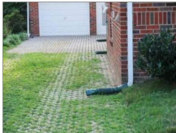
Figure 3-3: Downspouts directed to permeable pavement on driveway (courtesy of Montgomery County, MD)
