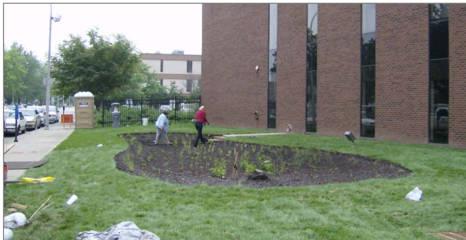
Figure 4-2: Picture of a rain garden under construction (courtesy of URS Corporation)
