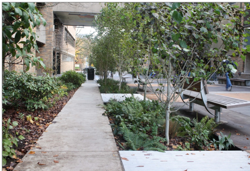
Figure 3-2: Disconnection at Portland State University, Oregon, where vegetated areas are distributed throughout the impervious courtyard area.
