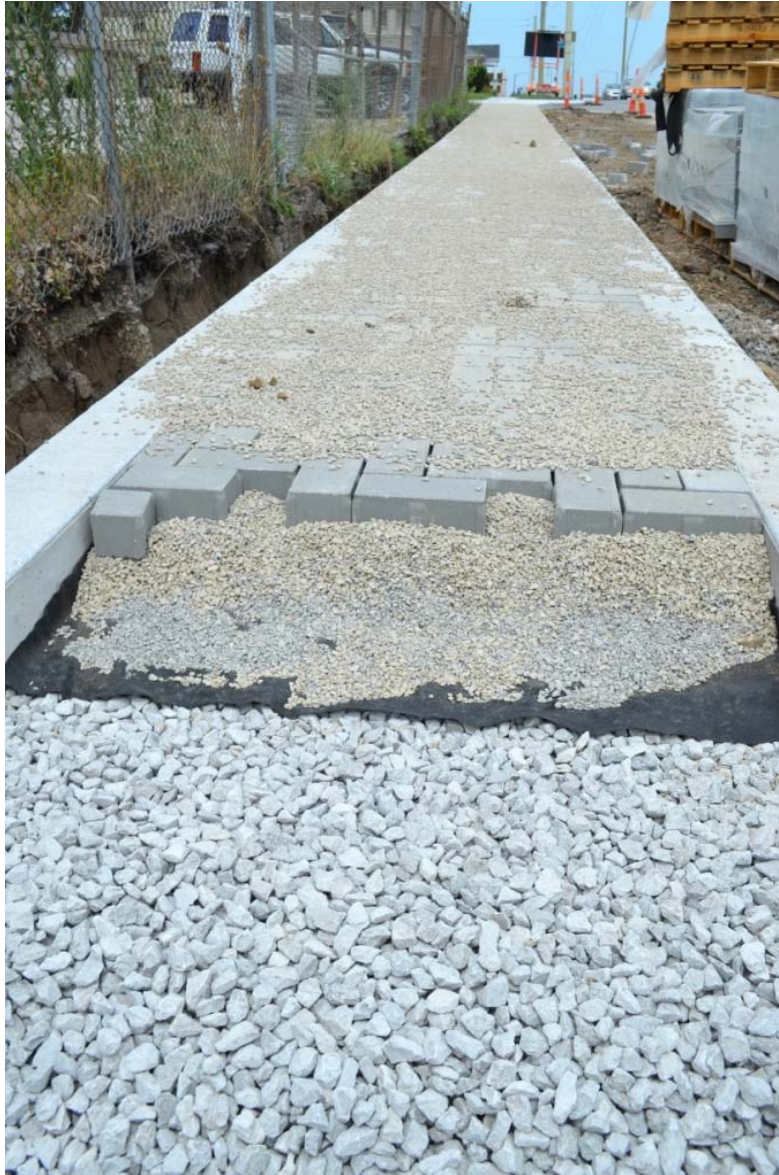
Figure 4-9: Porous pavement sidewalk installation with filter fabric placed beneath the gravel and stone layers (courtesy of URS Corporation).
