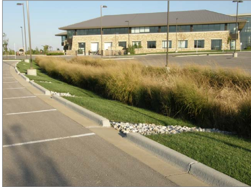
Figure 4-3: Picture of a bioretention facility (courtesy of David Dods)
