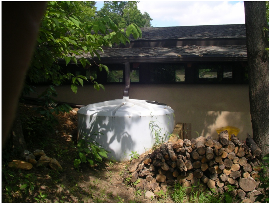
Figure 4-10: Picture of a rainwater collection system (courtesy of David Dods)
