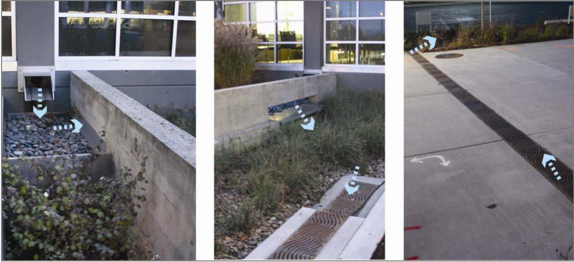
Figure 3-5: Treatment train approach: disconnected downspout runoff enters a series of vegetated controls.
