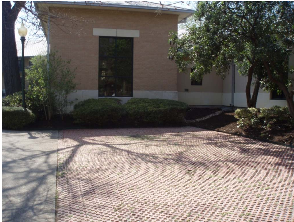
Figure 4-8: Picture of permeable pavers in portion of parking lot in San Antonio (courtesy of David Dods)
