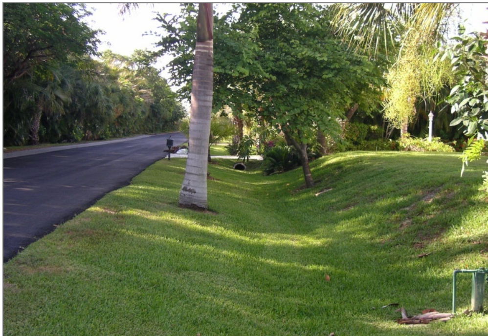
Figure 4-5: Picture of a typical swale (courtesy of David Dods)
