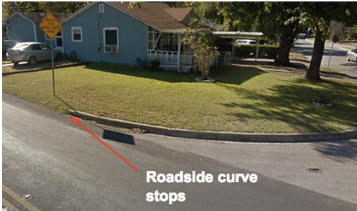
Figure 2: South side of 38th 1/2 Street Curb
