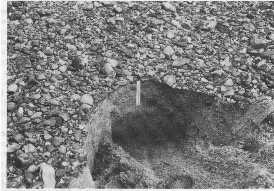
Figure 13-7. Static Armor layer below Fort Randall Dam (Livsey, 1963)
