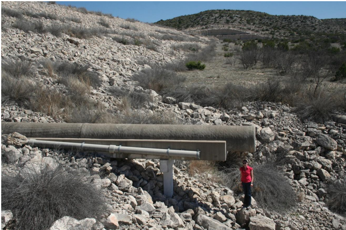
Figure 14 – Circular Conduit Outlet for Dam Site 10
