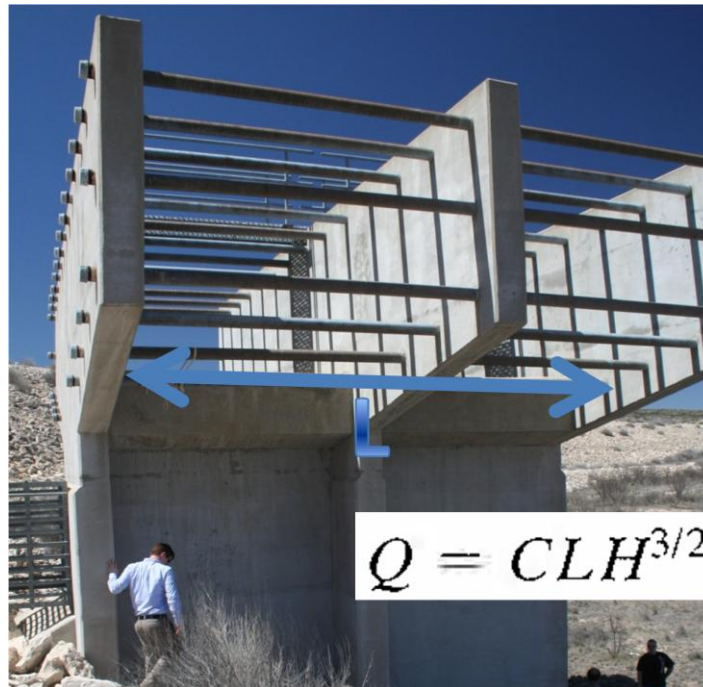
Figure 16 – Dam Site 11 Principal Spillway(2 nd Stage-Weir flow)
