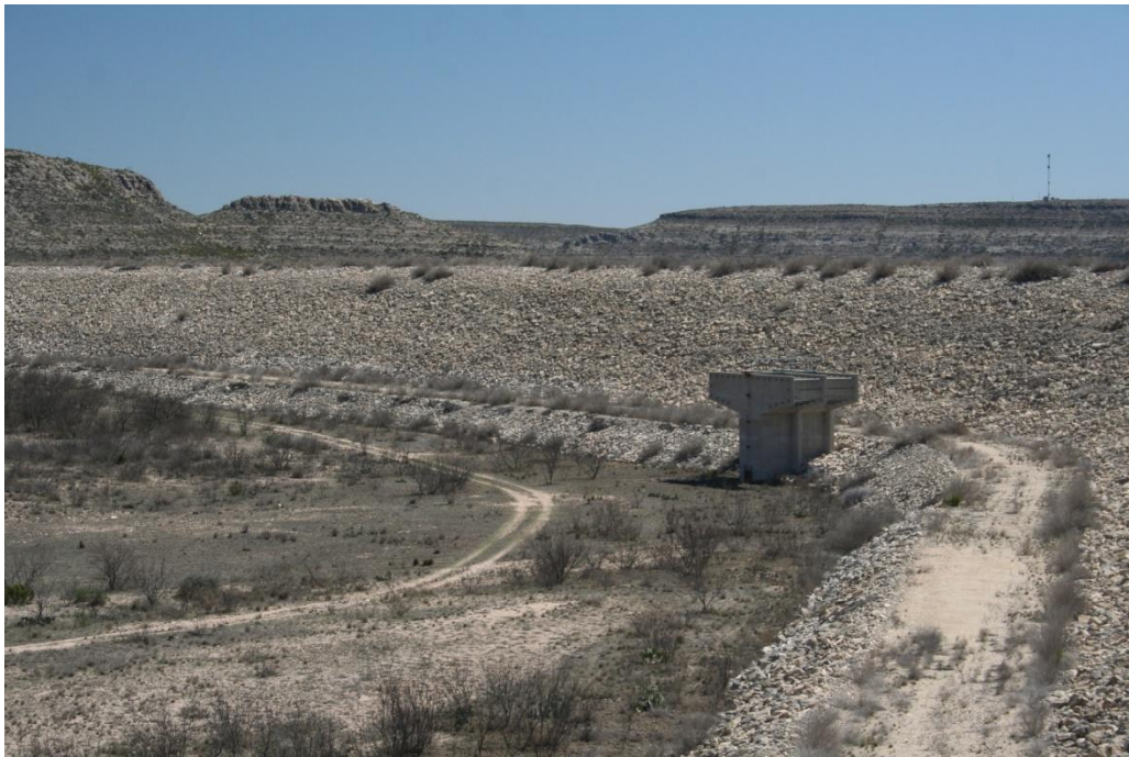
Figure 12 – Dam Site 11 Principal Spillway Structure
