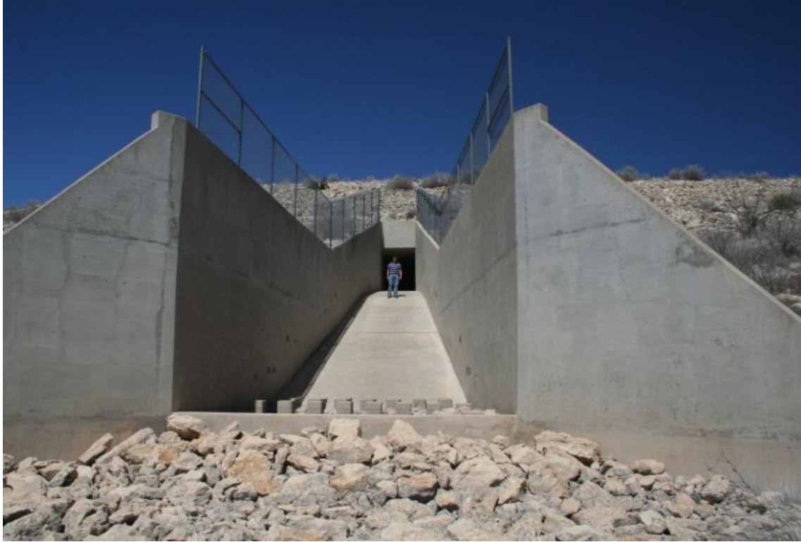
Figure 13 – Rectangular Conduit Outlet for Dam Site 11
