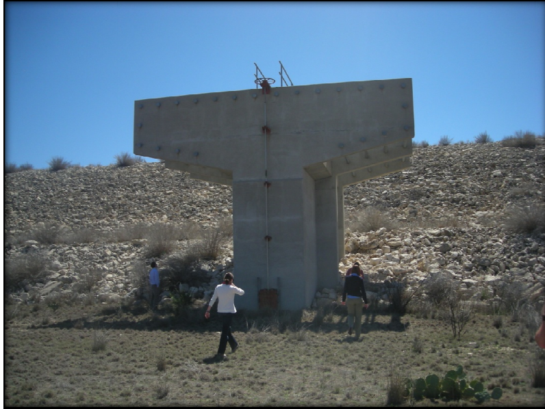
Figure 3: Principal outlet of the dam located in the site #11
