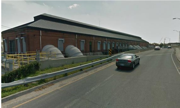
Figure 1: Old pumping station on Broad Street
