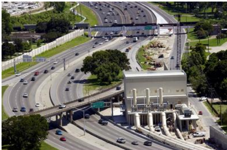
Figure 2: New pumping station off I-10
