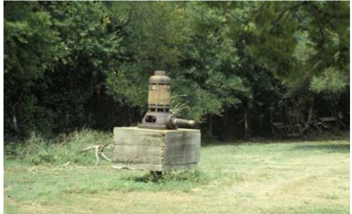
Figure 1: This pump in Baytown, Texas, was level with the surface of the ground when first installed. Image provided by John M Sharp, PhD., at the University of Texas at Austin.
