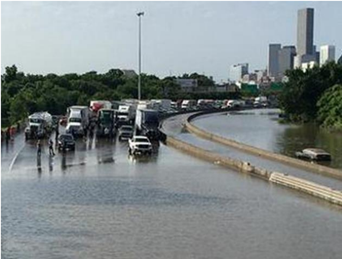
Figure 1. I-45 North blocked during Houston's Memorial Day 2015 flood event. 2
