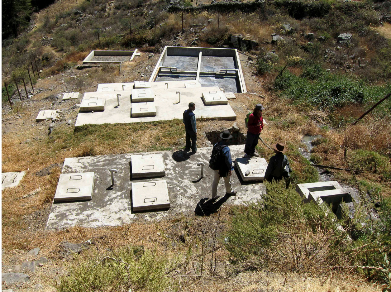
Huasta wastewater treatment plant
