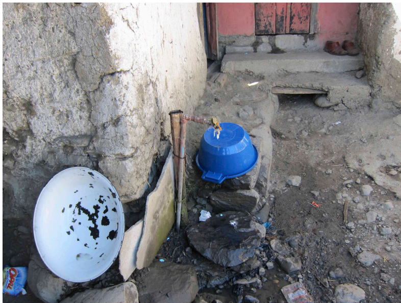
Water supply at Soledad President's house.
