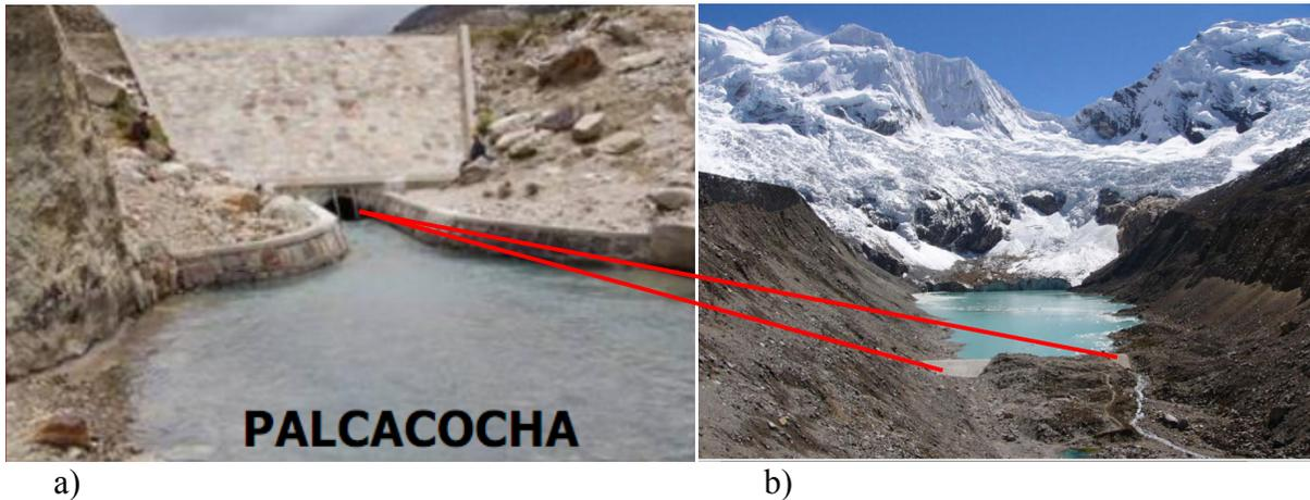
Figure 5: a) Hydraulic structures for draining water from Lake Palcacocha. b) Front view of the Lake in September 2004 showing the two artificial concrete dams (photo by Z. Patzelt 2004 cited in Vilimek et al. 2005).
