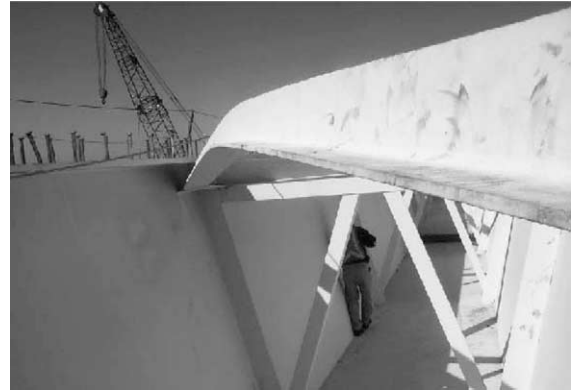
Fig. 2. Trapezoidal box girder failure during construction.
