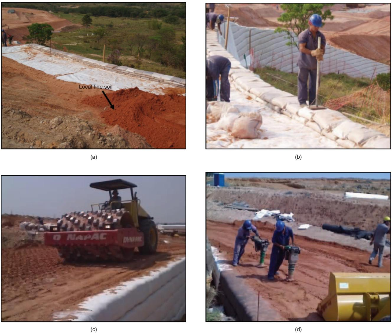
Figure 2. Compaction process: (a) soil spreading; (b) soil bag facing; (c) compaction roller; (d) hand-operated tampers
