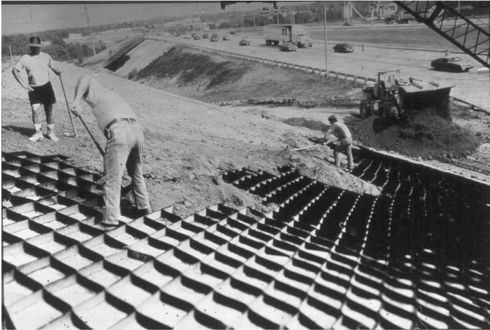
FIGURE 37.15 View of expanded geocell (photo courtesy of Presto Product Company).
