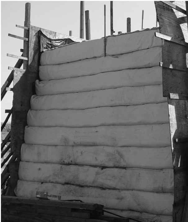
Figure 1 – Geotextile reinforced soil retaining wall
