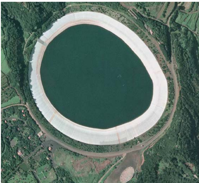
Figure 1. Aerial view of the “Laguna de Barlovento” reservoir, waterproofed with PVC-P geomembrane.
