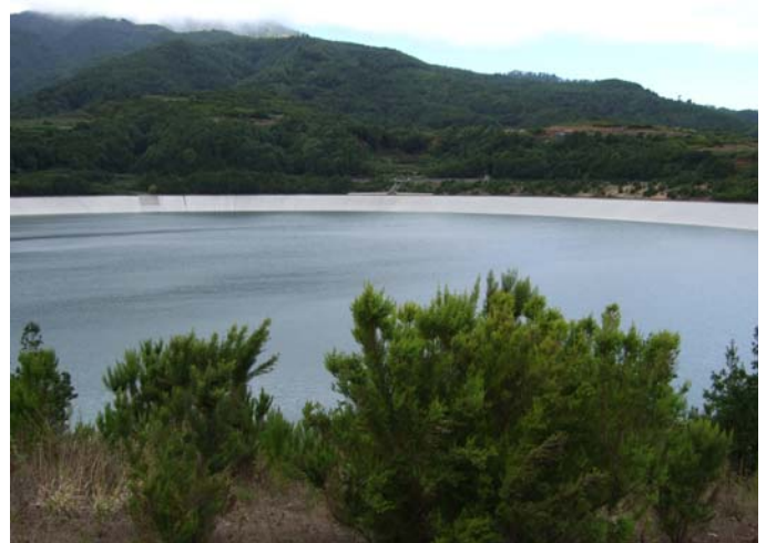
Figure 2. View of the geomembrane-lined reservoir.
