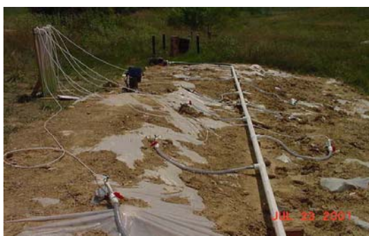
Figure 80. PV drains at the Columbia landfill site.
