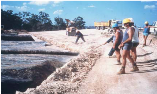
Figure 52. Geomembrane installation for shallow cut-off walls.
