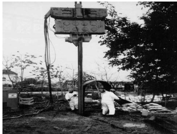
Figure 75. Installation of HDPE barrier wall utilizing conventional
