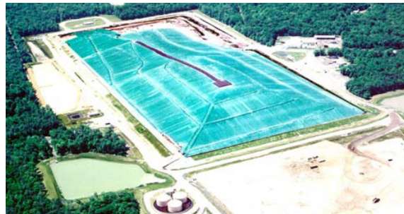
Figure 42. Exposed geomembrane cover over Cells 1 and 2 of the DSWA's southern facility.
