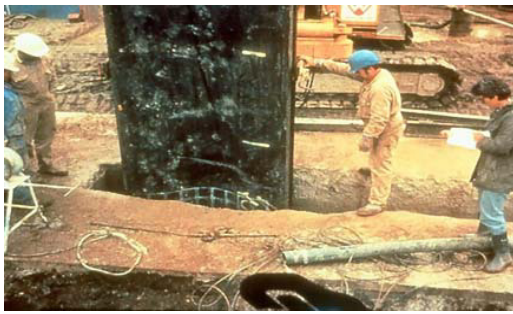
Figure 51. Geomembrane insertion in a dry trench.
