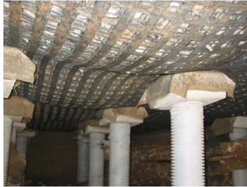
Figure 3: Pile Foundation with Geosynthetic Support
