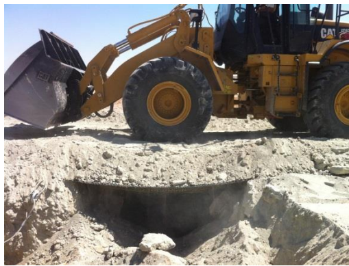
Figure 2: Void Bridging Test Section
