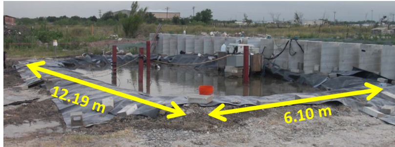
Figure 6: Inundation berm with four stand pipe piezometers behind the wall.
