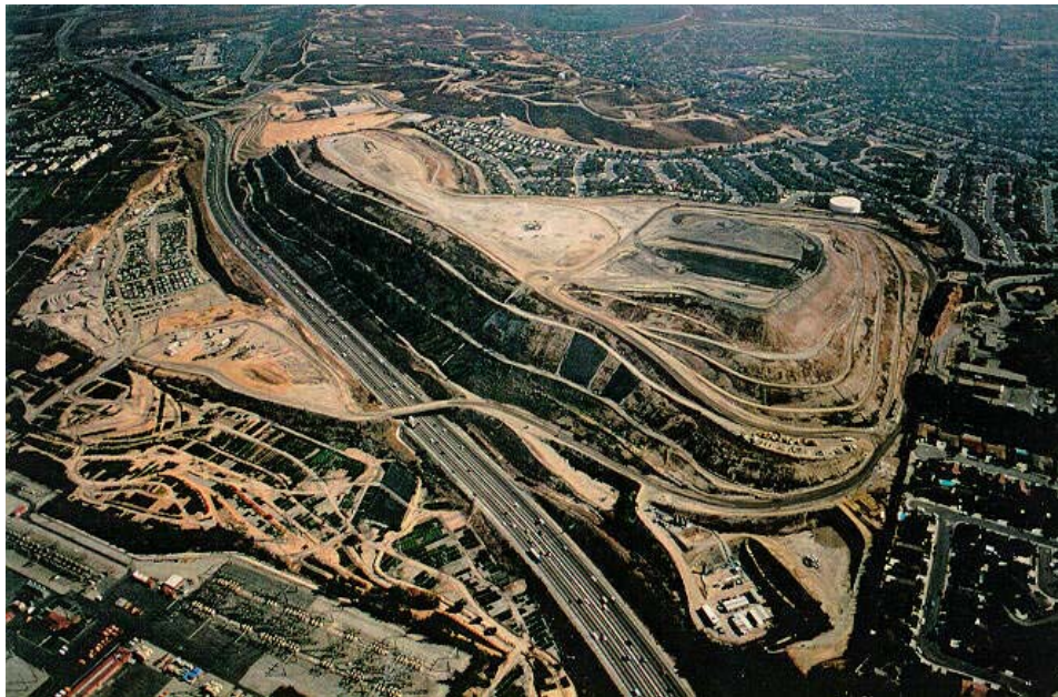
Fig. 2. View of OII Superfund Landfill Before Construction of the Evapotranspirative Cover System
