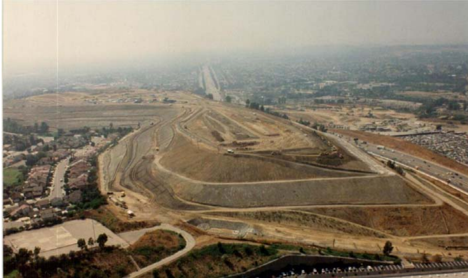
Fig. 3. View of OII Superfund Landfill shortly after Construction of Evapotranspirative Cover System
