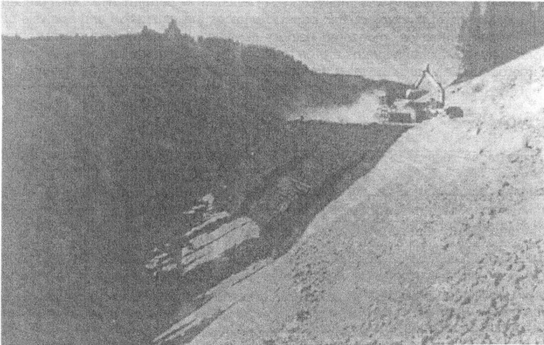
Figure 1. Finished reinforced slope with erosion matting in place.
