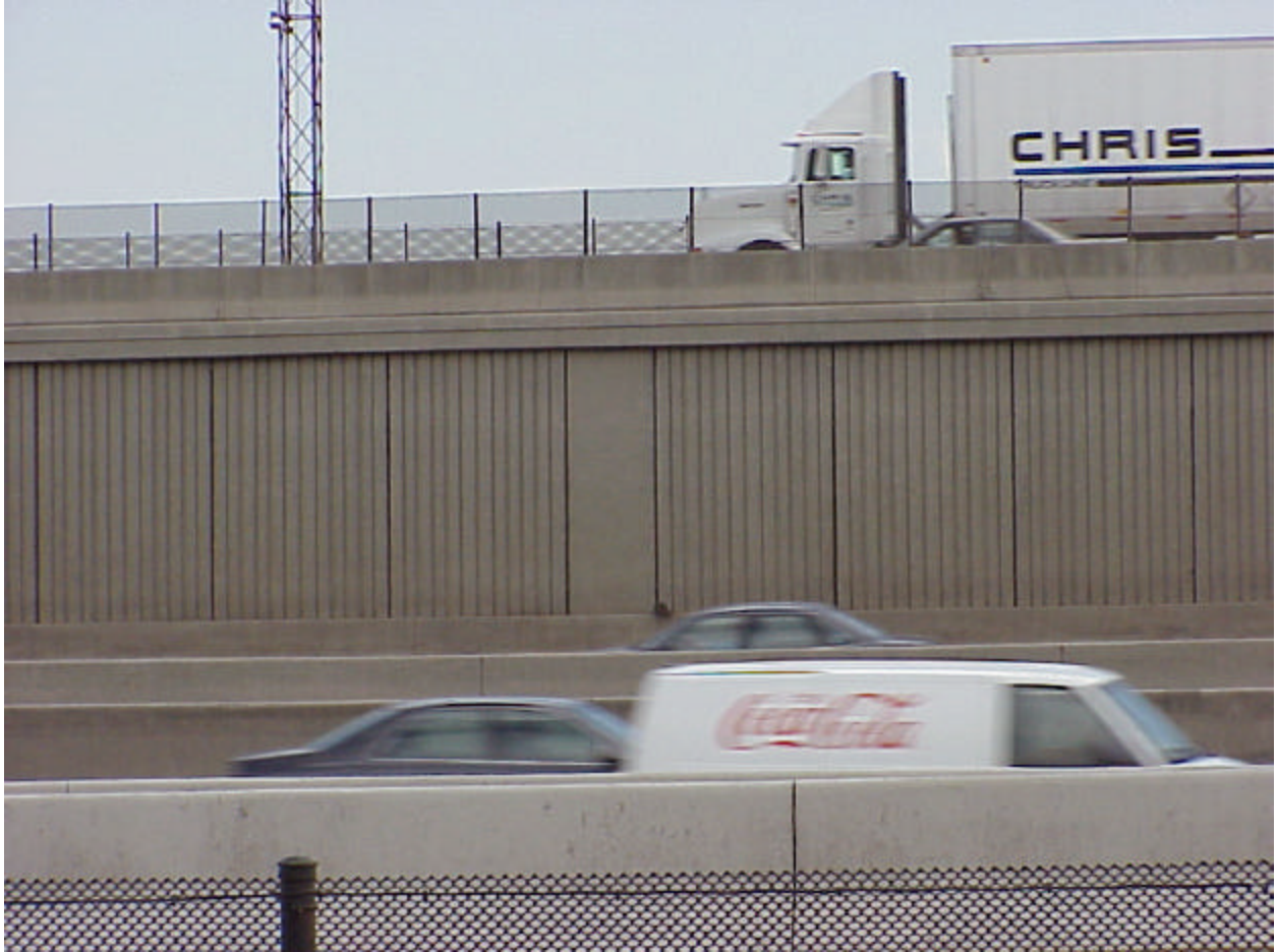
Figure 1.2. Picture of the Completed I-25/I-70 MSE Wall with Independent Full-Height Facing in Denver, Colorado.
