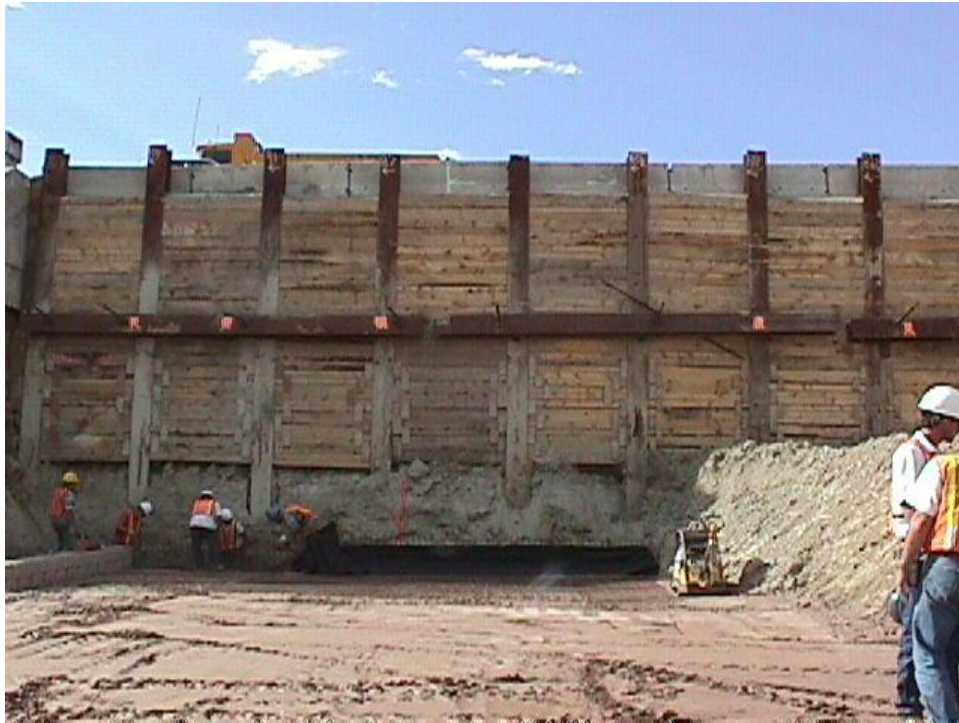
Figure B-17. The first layer of fill material at the east side of the Phase I Structure has been placed. In the background, H-beams and shoring support the approach to the old bridge during the construction of the Phase I Structure.
