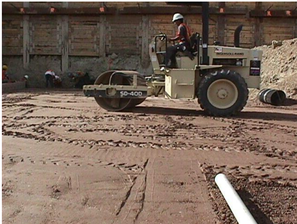
Figure B-21. A vibratory roller was used to compact the fill material.
