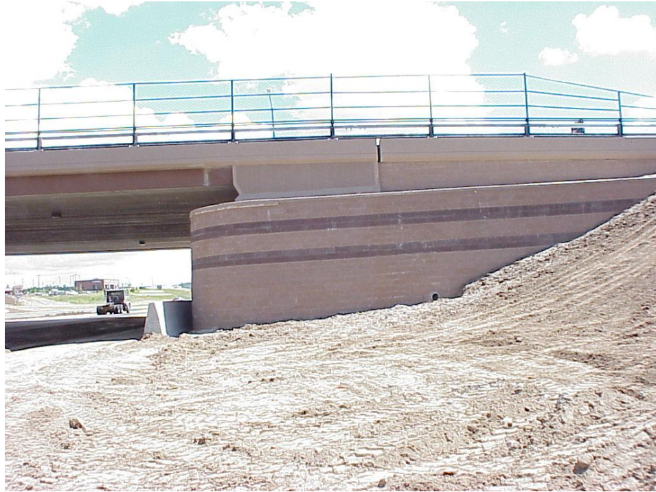
Figure B-1. A view of the northwest side of the completed Founders/Meadows bridge-approaching roadway structure showing lower and upper MSE walls, wing walls, and girders.
