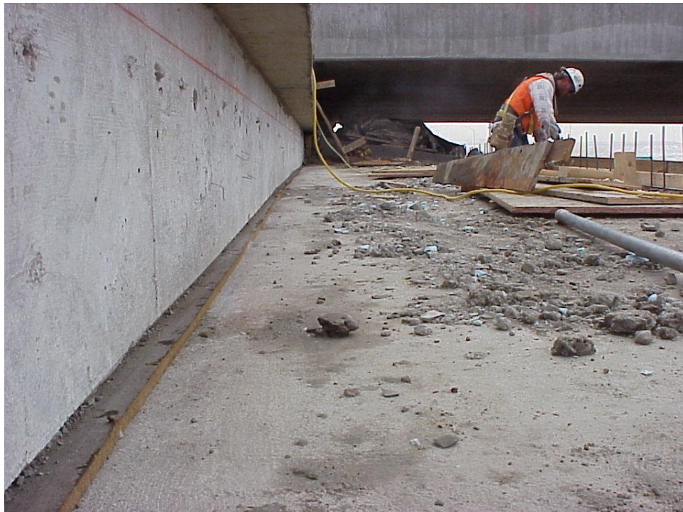
Figure B-28. Expansion joint material was installed below the sides of the abutment wall on top of the footing. In the center zone below the abutment wall on top of the footing, galvanized sheet metal centered on a bearing pad was placed (see figure 29).
