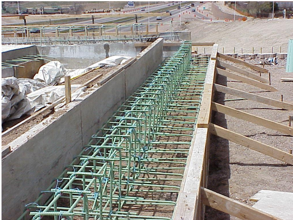
Figure B-42. The forms and reinforcing steel for the sleeper foundation supporting the approach slab.
