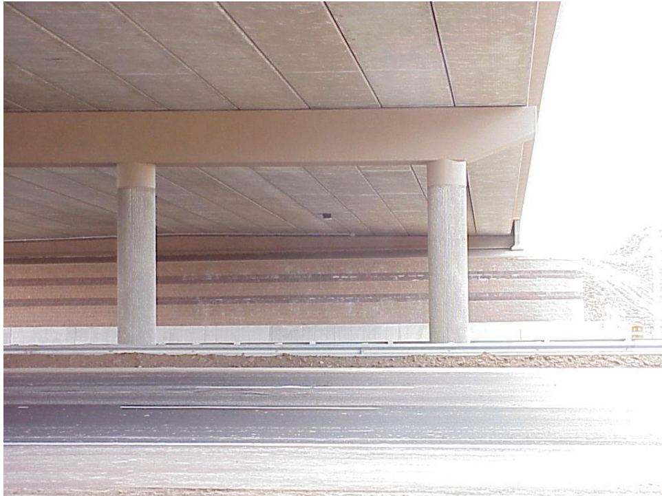
Figure B-2. A view of the east side of the Founders/Meadows Bridge showing front MSE wall, girders and pier columns.
