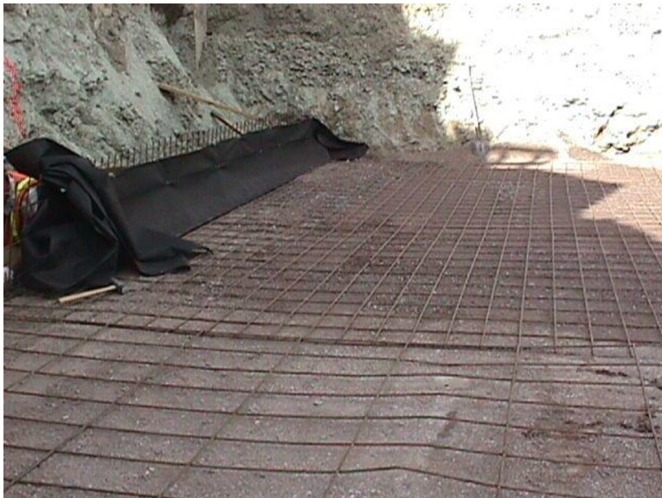
Figure B-18. The northern side of Phase I structure was internally stabilized with steel wire mesh. The steel extended past the edge of the wall and was tied to the geogrid placed to stabilize the front MSE wall.
