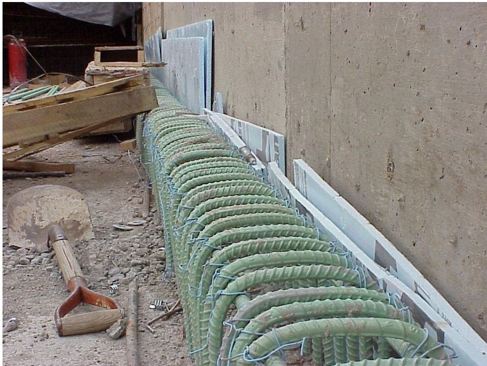
Figure B-32. A reinforced concrete “kicker” strongly attached to the bridge foundation was placed behind the bottom of the abutment wall. This kicker was placed to provide an extra bracing at the top of MSE wall for global stability.
