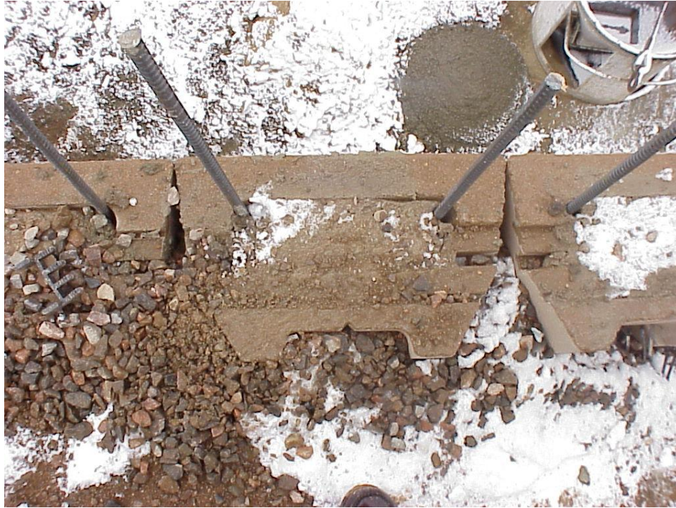
Figure B-27. The top two rows of blocks were filled with concrete. Steel rebar inserted in the plastic concrete were later bent over to tie the concrete cap at the top of the front MSE wall.
