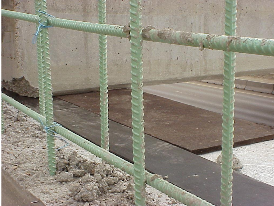
Figure B-31. The elastomeric bearing pad and expansion joints material placed on the abutment wall where girders will be seated.
