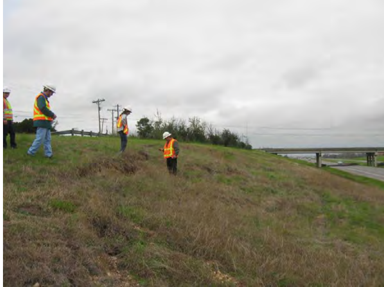
Figure D.31 Vertical extent of separation at the scarp
