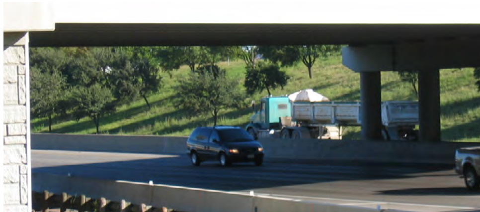
Figure D.2 Embankment 1 looking from Embankment 3
