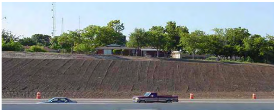
Figure D.37 Original slope after remediation with tire bales. (TXDOT)
