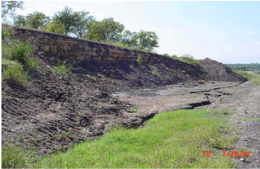
Figure D.39 Failed Slope 2001
