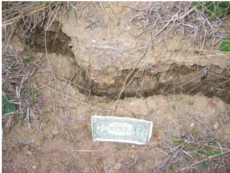
Figure D.36 Close-up of lateral crack cutting through the center of the failed mass
