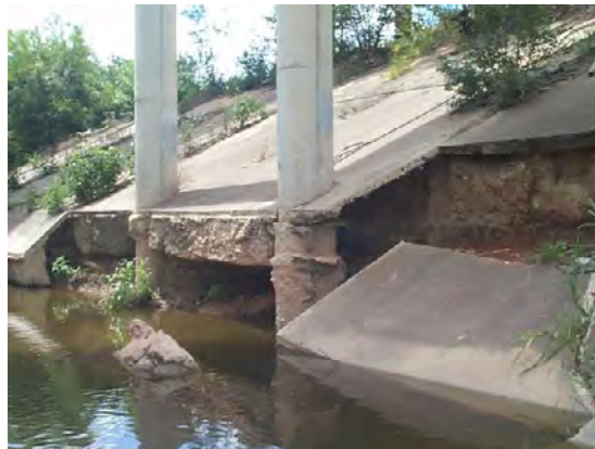
Figure D.23 Partially exposed foundation (South foundation 1999*)
