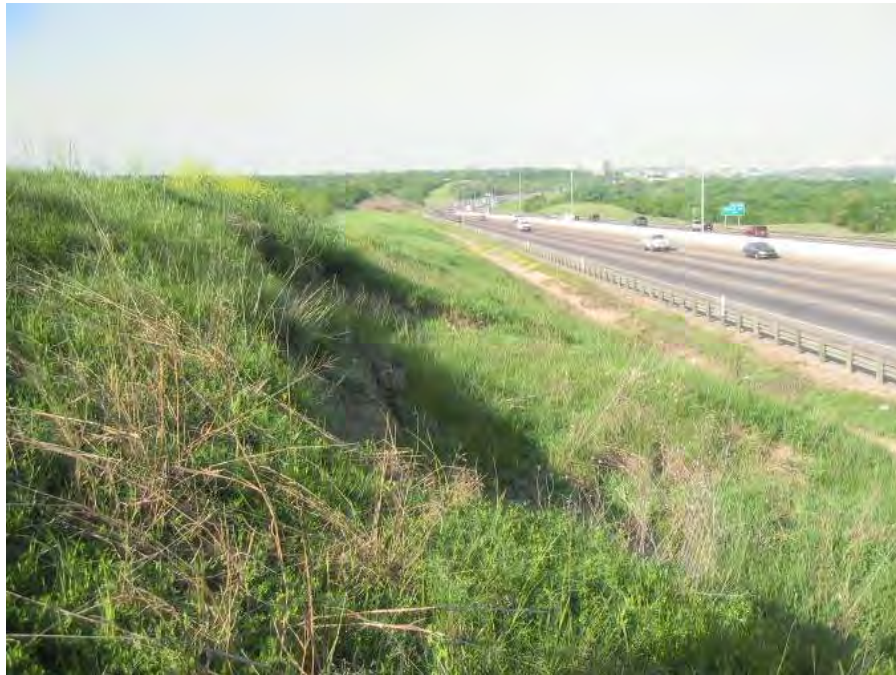
Figure D.50 Adjacent slope failure 2005
