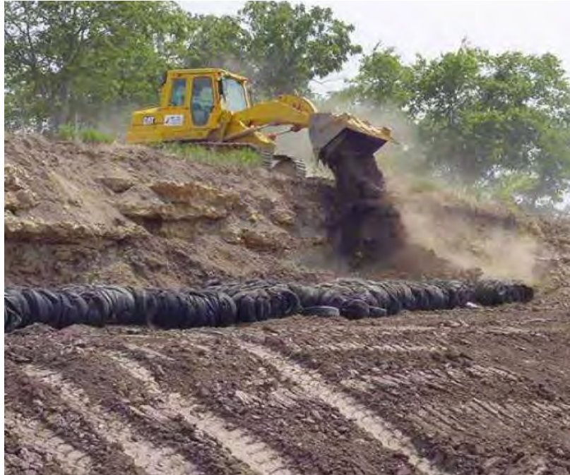
Figure D.43 Placement of soil layer 2001
