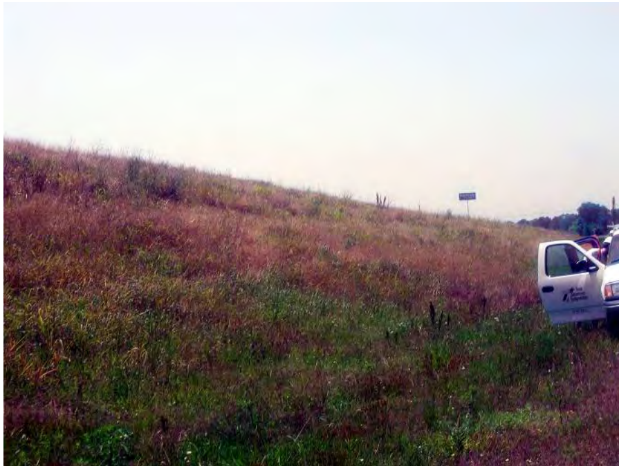
Figure D.61 Side View of the Southwest Embankment at the Intersection
