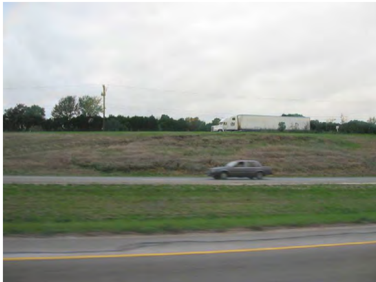
Figure D.32 Lateral extent of slope failure
