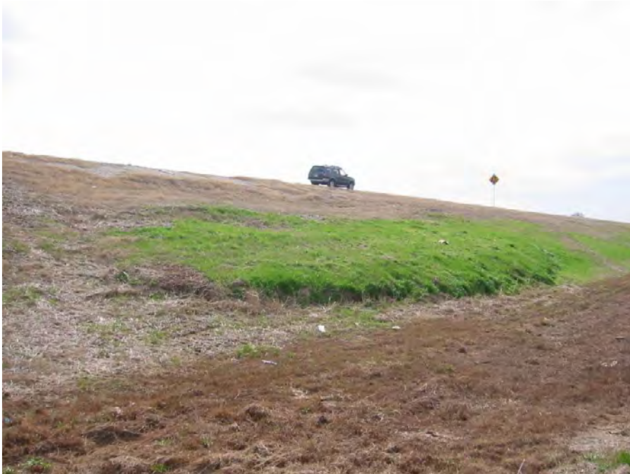
Figure D.64 View of failure facing eastward
