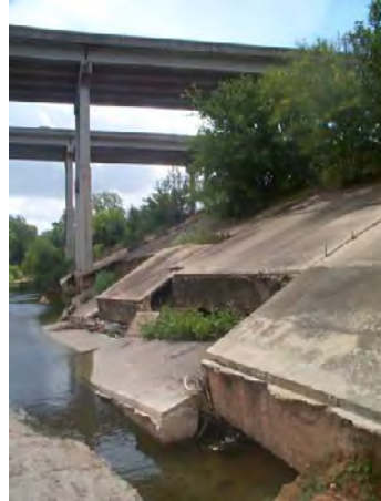
Figure D.17 Concrete facing (Southwest bank 1999*)
