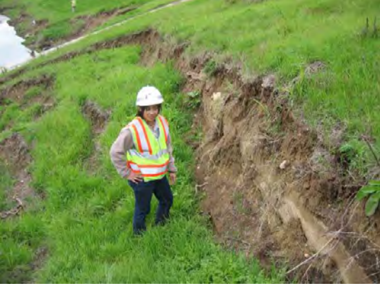
Figure D.24 Gravity retaining structure (Northwest - eastward 2005)
