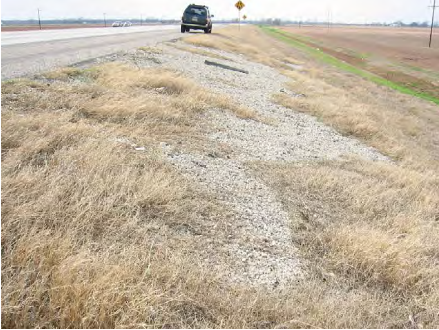
Figure D.65 View of remedial efforts at scarp of slide
