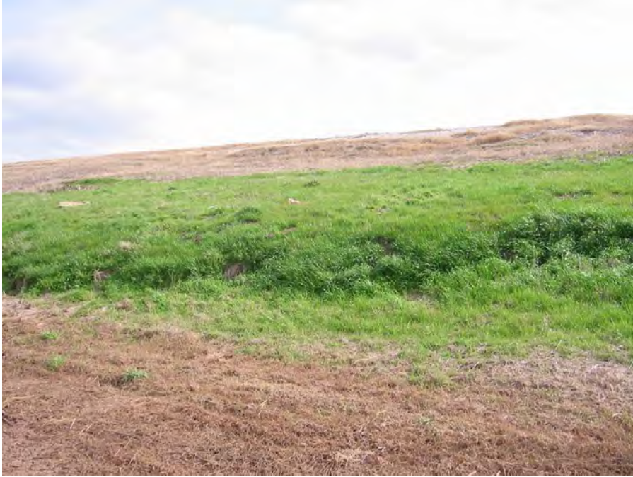
Figure D.63 View of toe bulge facing the slope
