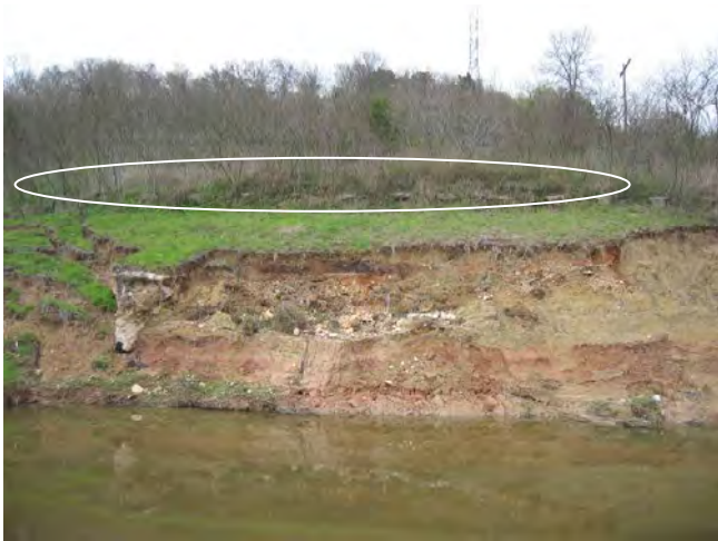
Figure D.20 Drilled shafts (Northwest bank 2005)
