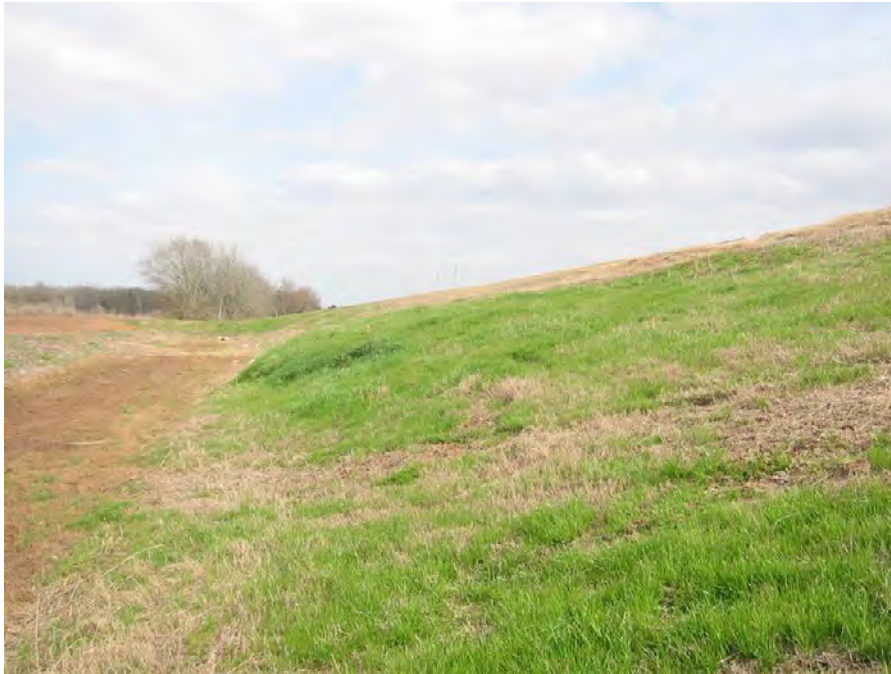
Figure D.62 View of toe bulge facing westward
