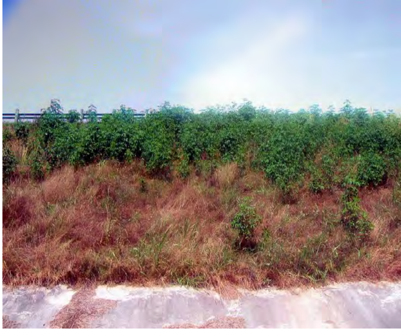
Figure D.60 Uphill View of Vegetation on Southeast Embankment.
