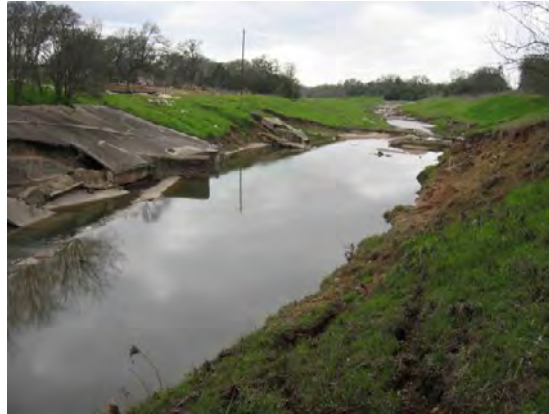
Figure D.29 Failing slope faces (Upstream view - westward 2005)
