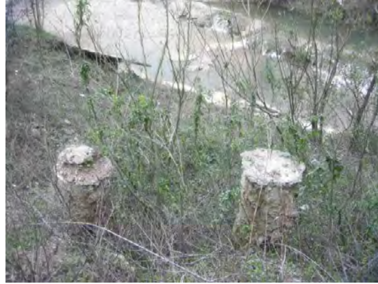
Figure D.25 Exposed drilled shafts (Northeast - southward 2005)
