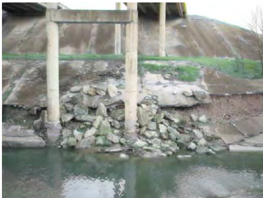
Figure D.22 Exposed foundation with rip-rap (South foundation 2005)
