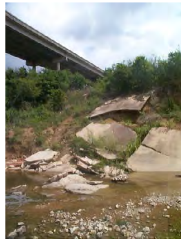
Figure D.19 Failing concrete cover (Northeast bank 1999*)
