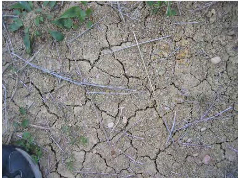
Figure D.34 Pattern of cracking within on the top of the failed mass
