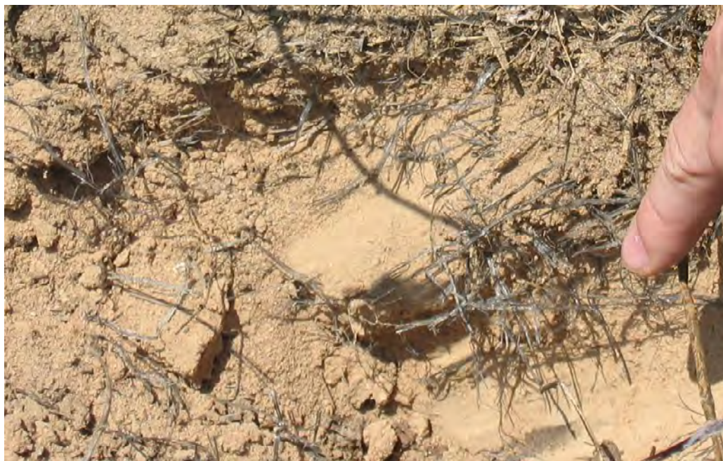
Figure D.53 Randomly Distributed Fibers in the Top Few Inches of the Embankment
