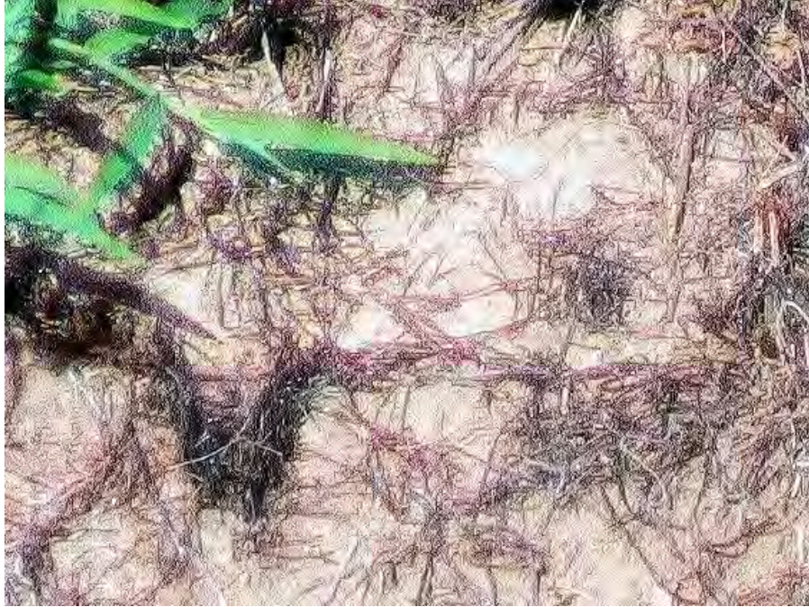
Figure D.58 Plan View of Embankment Surface; Notice that there are not any Visible Desiccation Cracks.
