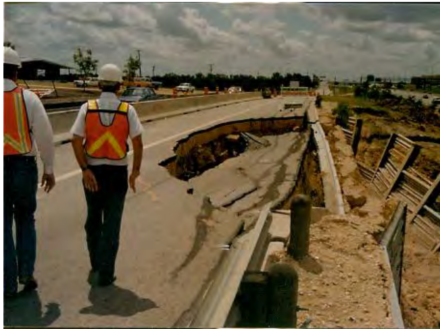
Figure D.6 Quadrant 4 looking South
