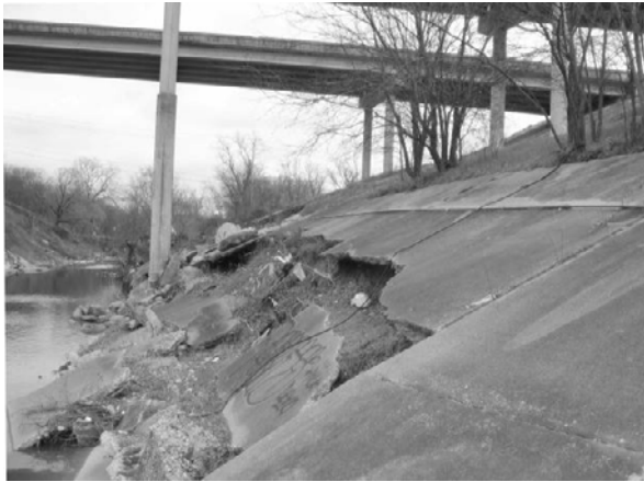
Figure D.16 Concrete facing (Southwest bank 2005)
