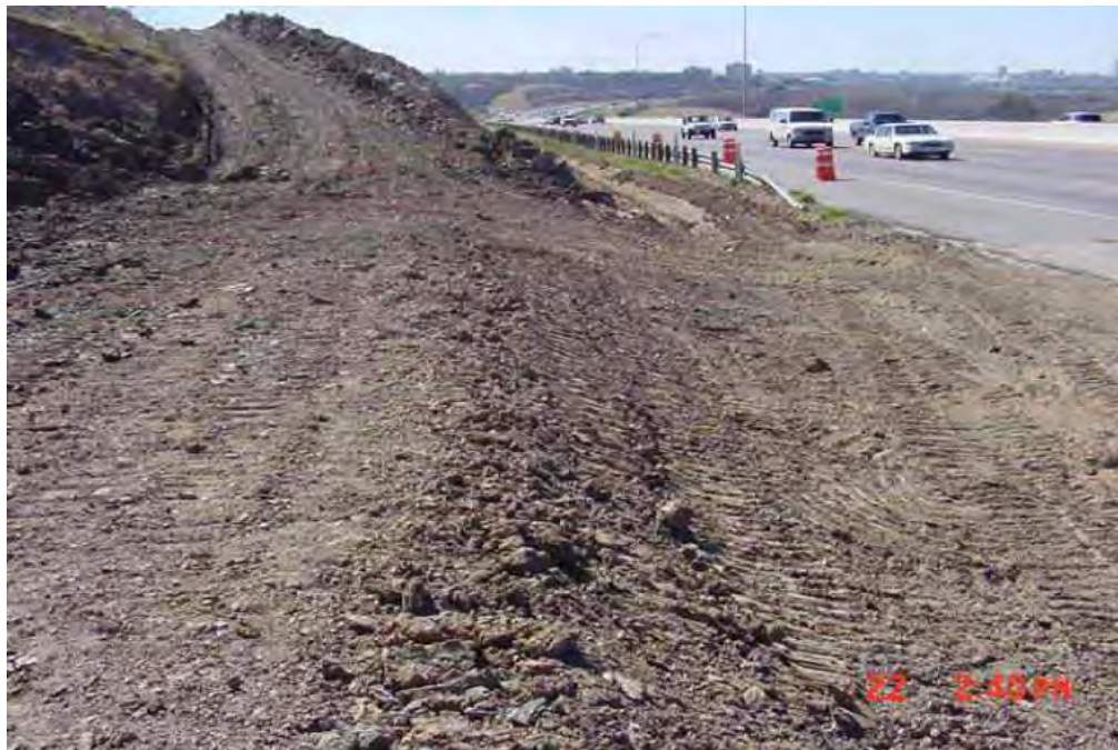
Figure D.44 Compacted soil layer 2001
