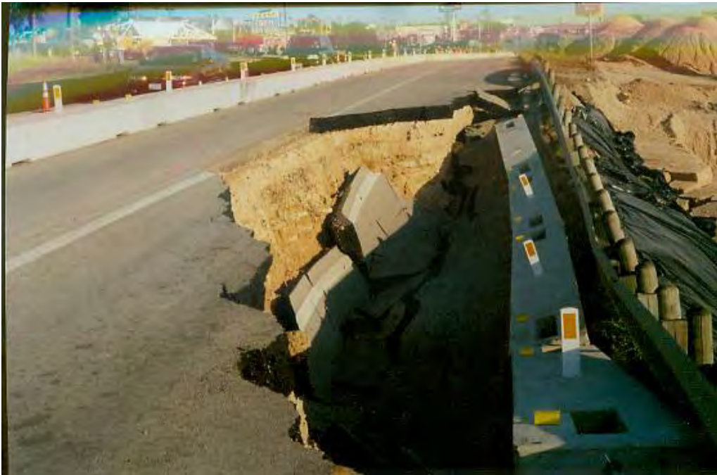
Figure D.8 Quadrant 4 looking South
