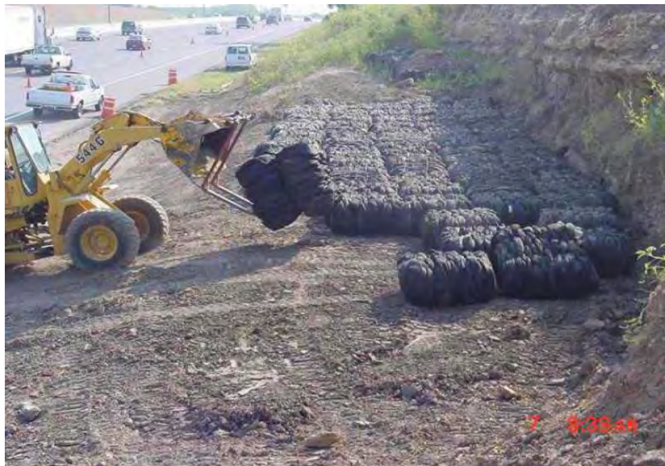
Figure D.42 Placement of first layer of tire bales 2001
