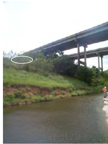
Figure D.21 Drilled shafts (Northwest bank 1999*)
