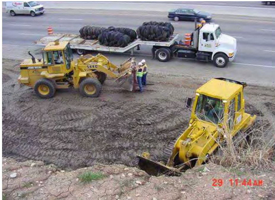
Figure D.41 Foundation preparation 2001
