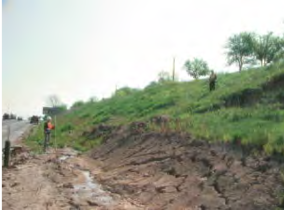
Figure D.47 Adjacent slope failure 2005
