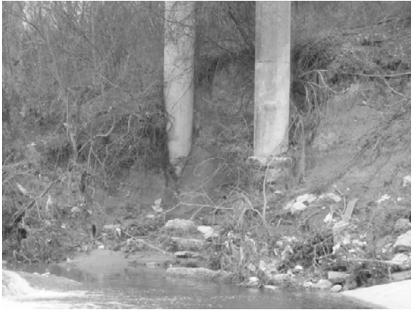
Figure D.26 Exposed foundation (North foundation 2005)
