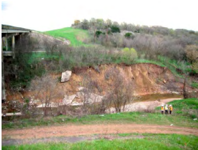
Figure D.18 Failed concrete cover (Northeast bank 2005)
