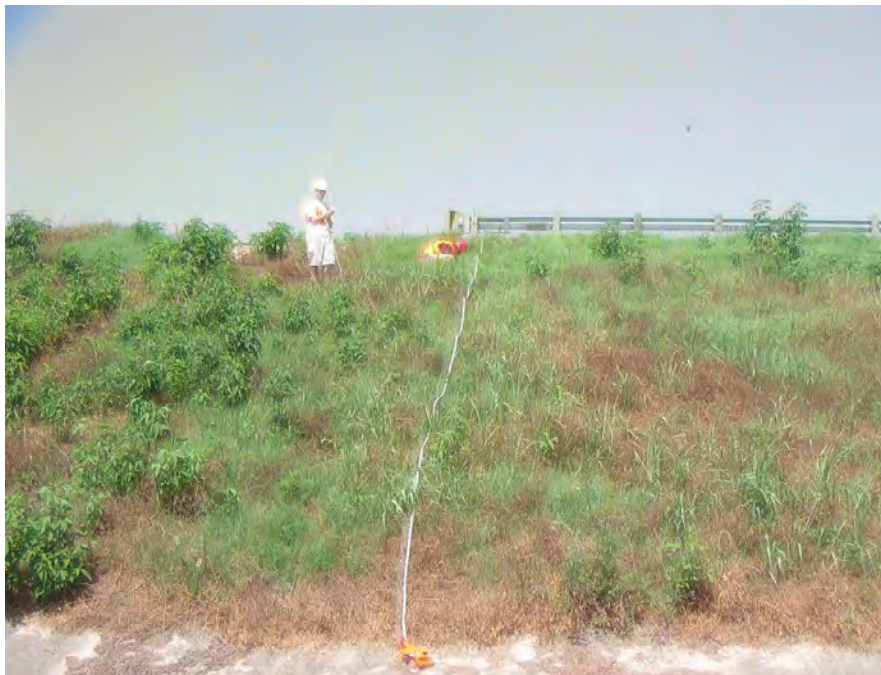
Figure D.59 Side View of Embankment on Southeast Side of Intersection.
