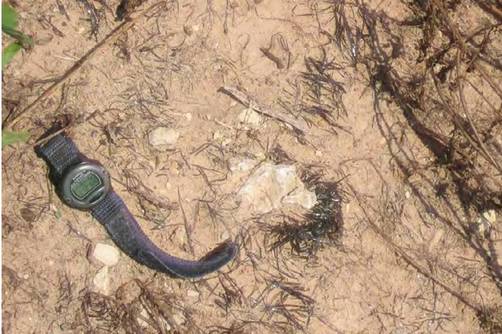
Figure D.54 Clumps of Fiber Reinforcement Located at Surface of Embankment
