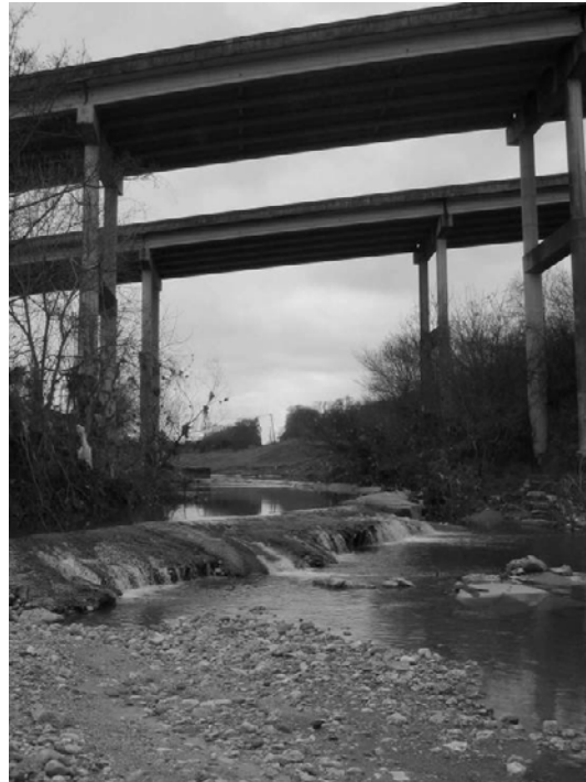
Figure D.15 Abandoned sewer pipe (Upstream view - westward 2005)
