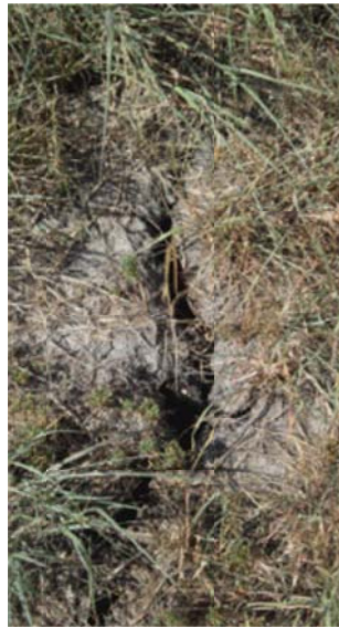
FIGURE 15 – Picture of Soil Cracks in Eastern Portion (Picture From Site Visit)
