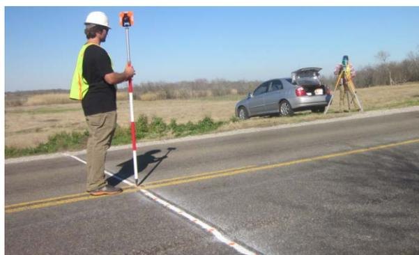
**Fig. 6.** Using total station and prism to monitor vertical deformations of the marked transverse sections
