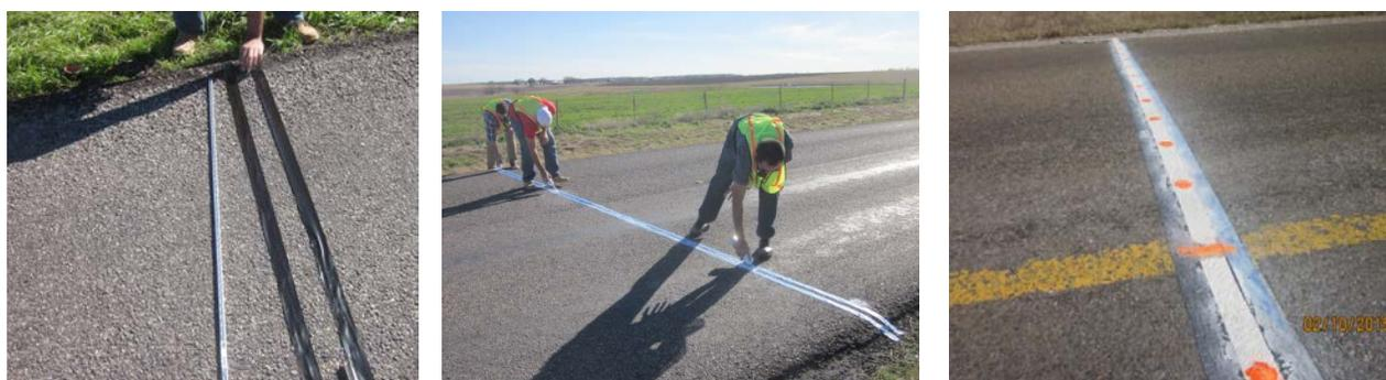
**Fig. 5.** Marking transverse test sections: (a) marking a stripe with duct tape; (b) painting the stripe with white spray paint; (c) painting circular orange marks on the white stripe
