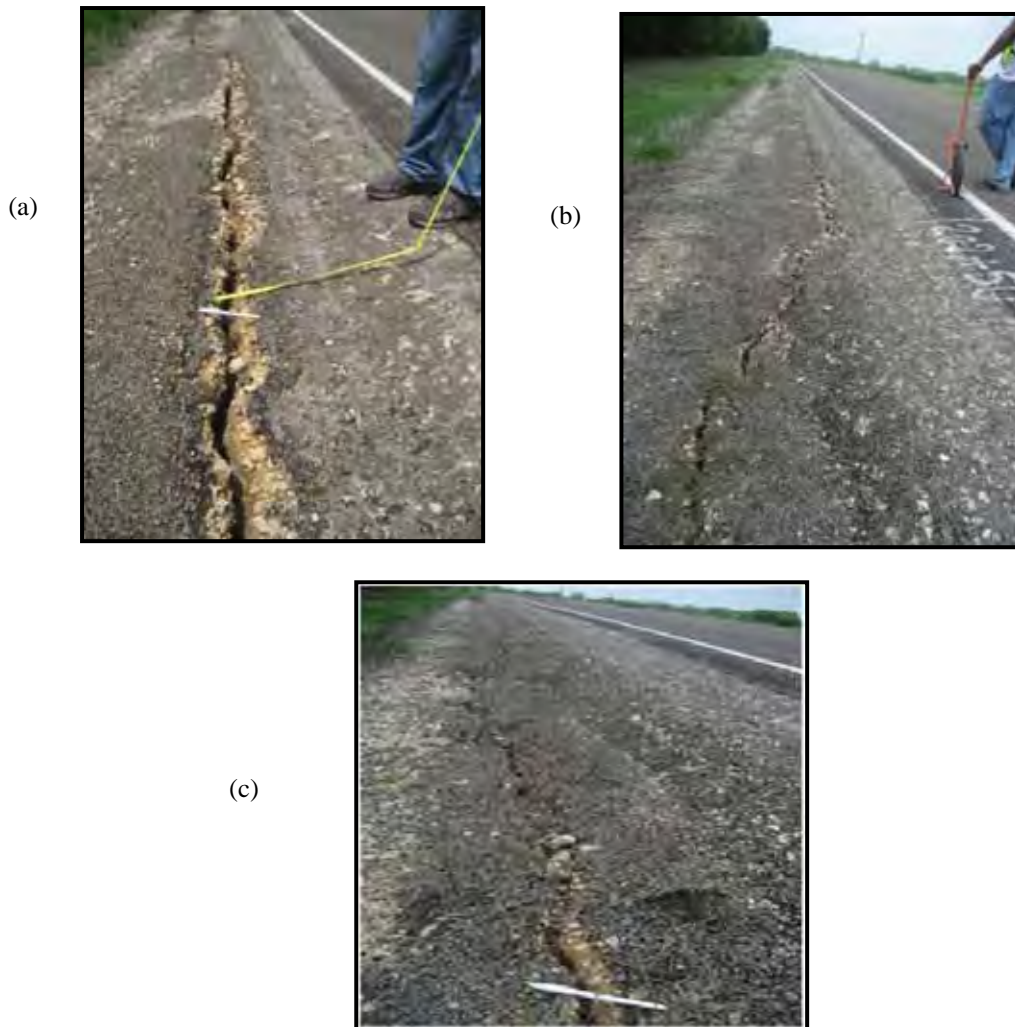
Figure 6.25: Typical cracks observed for sections with lime treatment and reinforcement. Date: August 2008
