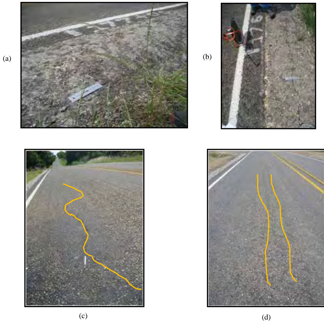
Figure 6.24: Cracks observed in Section 4Wb (#12)–No lime and PP geotextile. Dates: (a) April 2008; (b) August 2008; (c) May 2009
