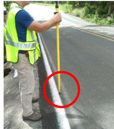
Place GPS unit on the road edge, at the level of the road pavement
