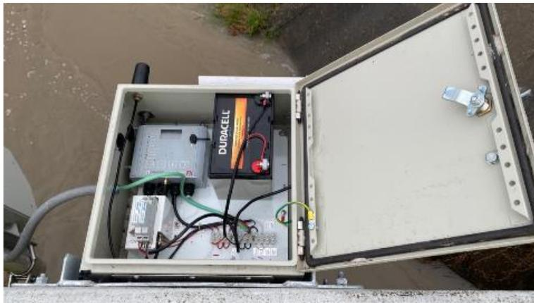
*Figure 3.2.2. Equipment housed in the gauge enclosure*
