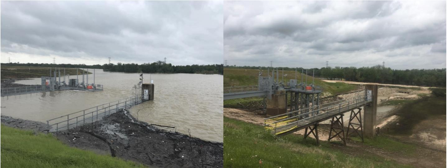
Figure 3: Addicks Reservoir during Hurricane Harvey on August 29th, 2017 with reservoir level at 108.8 feet. The image on the right shows the Addicks Reservoir during normal operation at a height of 69.45 feet on April 26th, 2018.<sup>8</sup>
