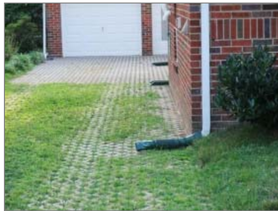
Figure 3-3: Downspouts directed to permeable pavement on driveway (courtesy of Montgomery County, MD)
