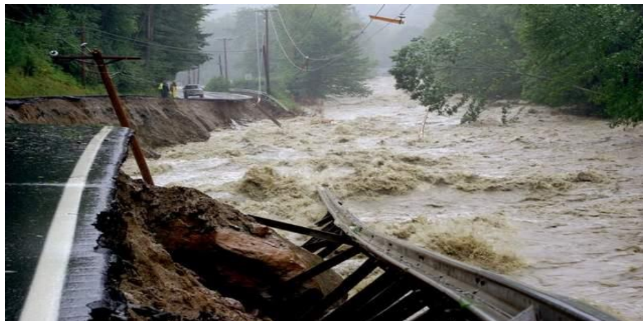
Figure 3. Picture of a roadway ripped off by Connecticut River in Vermont 2011
