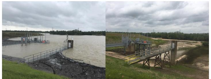
Figure 3: Addicks Reservoir during Hurricane Harvey on August 29th, 2017 with reservoir level at 108.8 feet. The image on the right shows the Addicks Reservoir during normal operation at a height of 69.45 feet on April 26th, 2018.8
