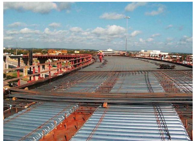
Fig. 6. Permanent metal deck forms (PMDF) and reinforcement installation.
