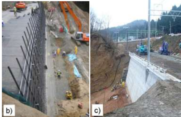
Figure 15: Railway embankment that collapsed during the 2004 Niigata-ken Chuetsu Earthquake and its reconstruction to a GRW RW having a FHR facing; a) cross-sections before and after failure and after reconstruction; b) wall during reconstruction; and c) completed wall (Morishima et al., 2005).
