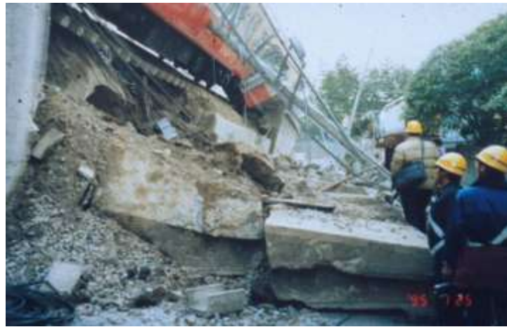
Figure 12: Gravity type retaining wall without a pile foundation at Ishiyagawa that collapsed during the 1995 Kobe Earthquake (Tatsuoka et al., 1996, 1997b).
