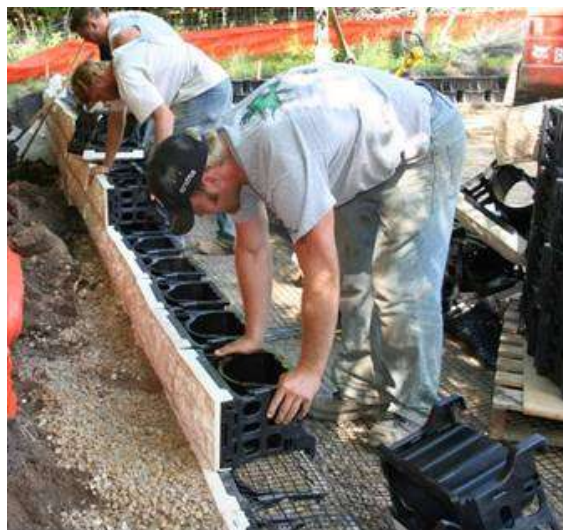
Figure 21: Construction of GRS wall with geosynthetic modular "block" units (courtesy Robert Race).
