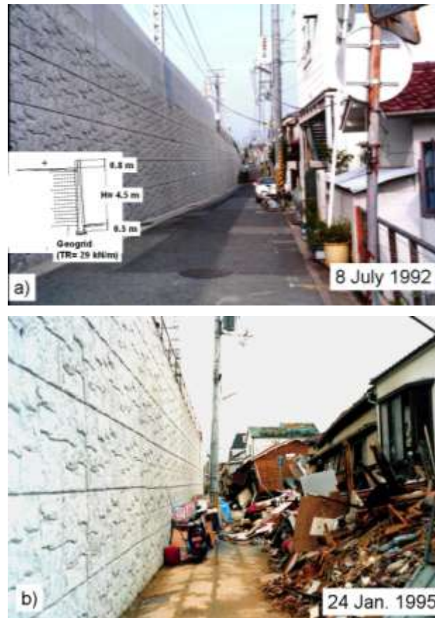
Figure 14: GRS RW having a FHR facing at Tanata, Japan; a) immediately wall completion; and b) immediately after the 1995 Kobe Earthquake (Tatsuoka et al., 1996, 1997b).
