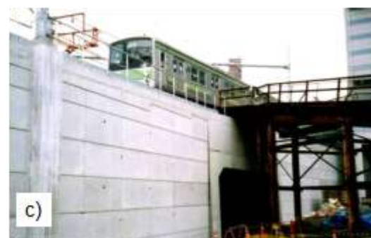
Figure 7: GRS RW having a FHR facing supporting one of the busiest rapid transits in Japan (Yamanote Line), near Shinjuku station, Tokyo (constructed during 1995 – 2000): a) typical cross-section; b) wall under construction; and c) completed wall
