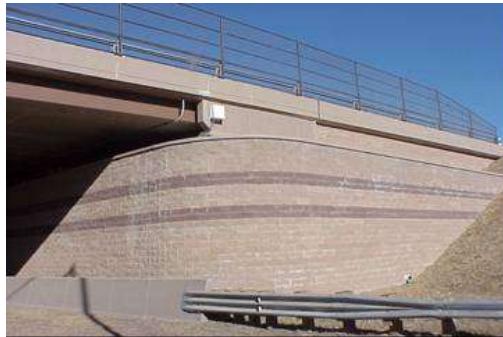
Figure 22: Founders/Meadows GRS bridge abutment.
