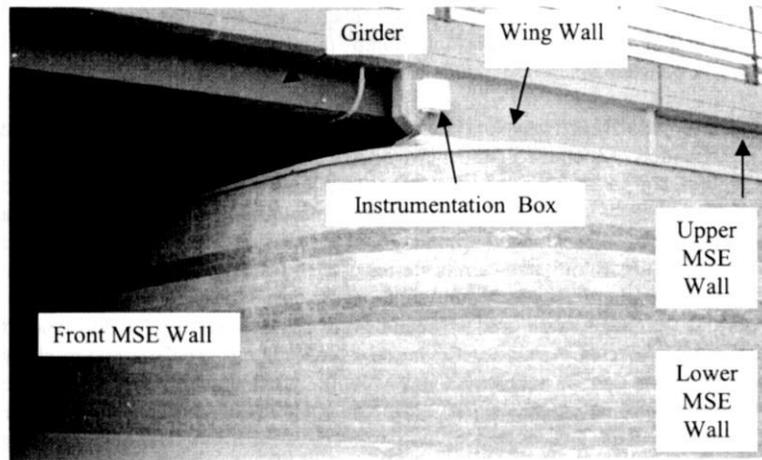
Fig. 1. View of the South-East Side of the Completed Founders/Meadows Bridge
