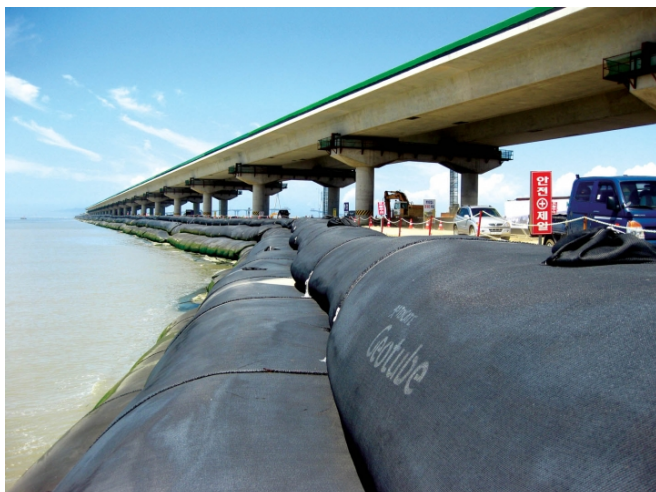
Fig. 6. Geotextile tubes for the construction of an artificial island at Incheon Grand Bridge Project, Korea (IFAI 2011)
