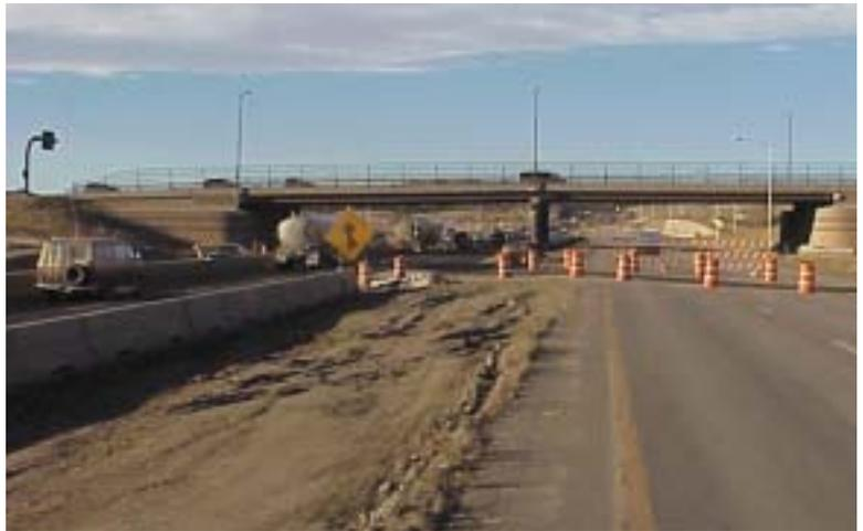
**Photo 1:** The Founders/Meadows bridge supported by GRS bridge abutments.
