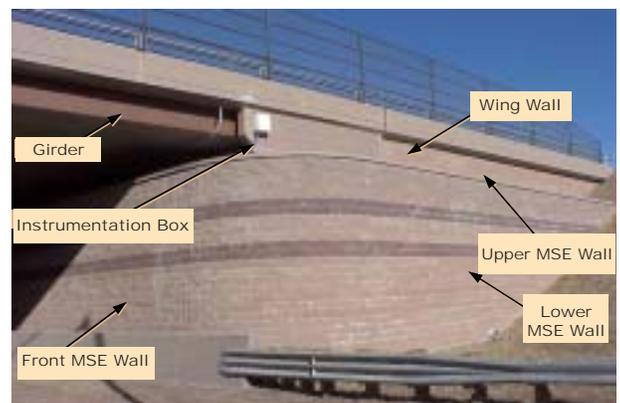
**Photo 2:** SRW components of a completed bridge abutment.
